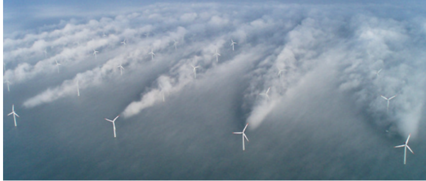
Figure 1: Wake effect on Horns Rev 1 wind park. Many offshore wind parks operating today are still on a regular grid, and so largely affected by wake effect. Source: [21]
